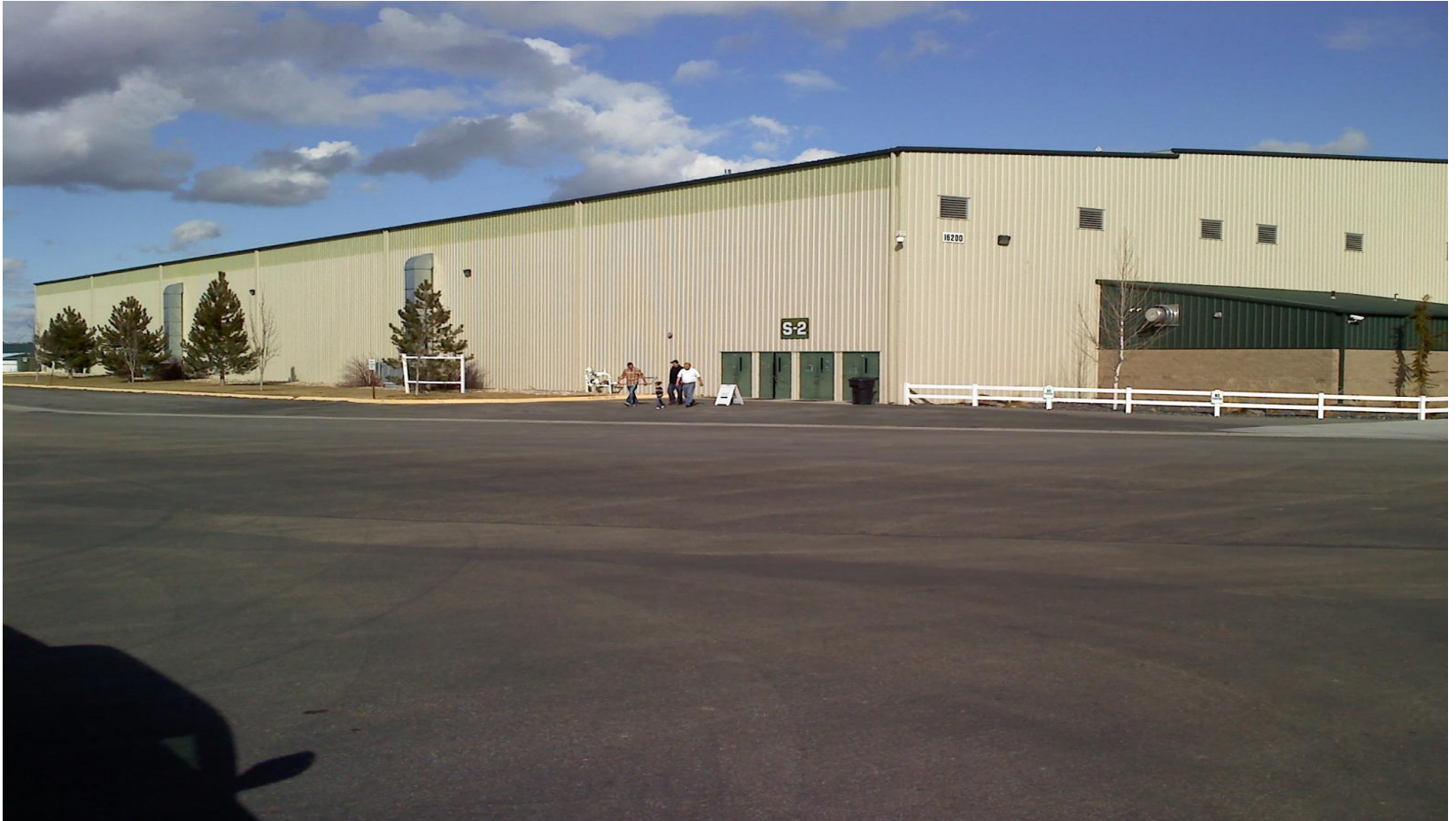
Boise state Jackson center indoor facility
