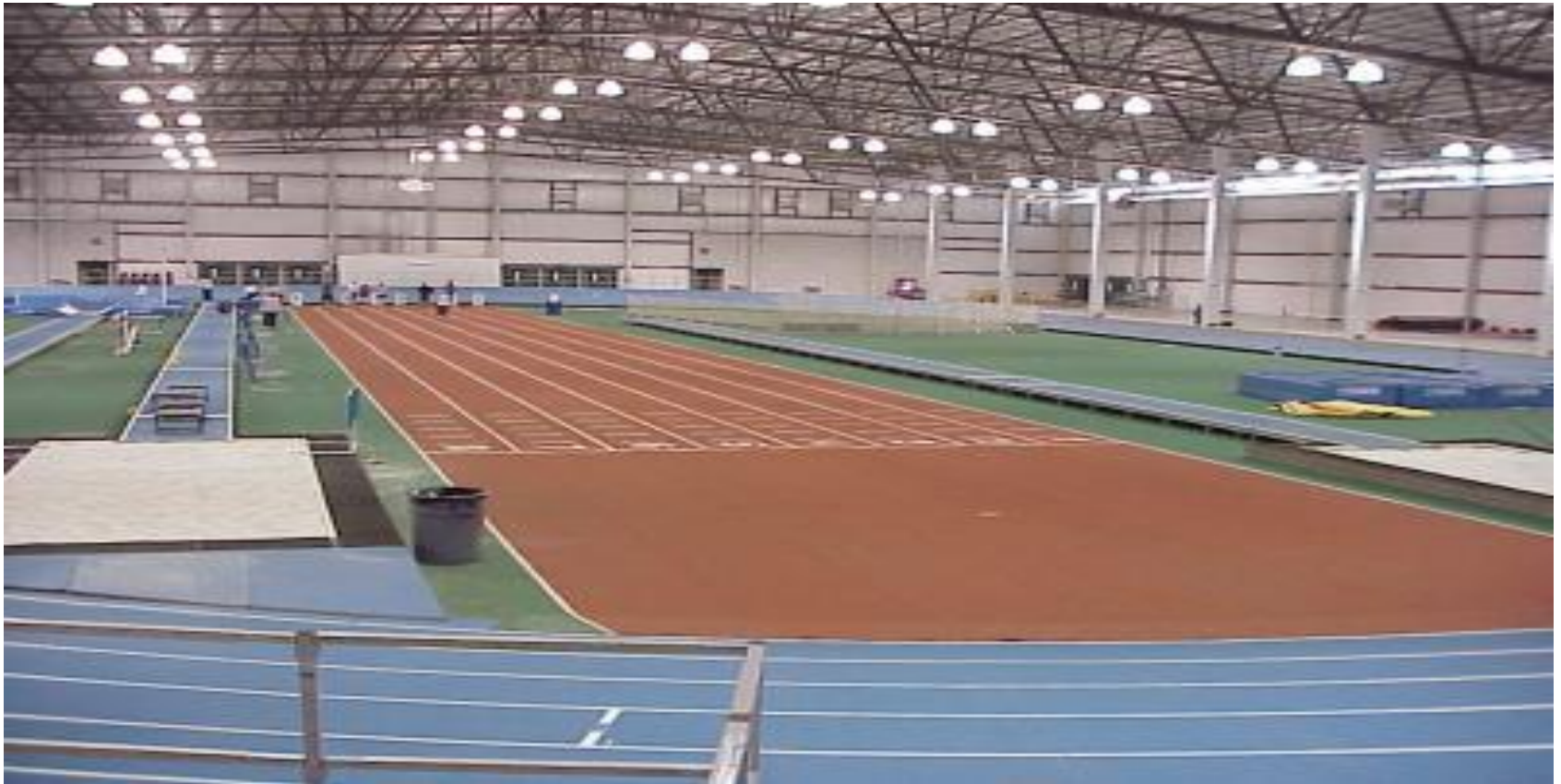
Boise state Jackson center indoor facility
